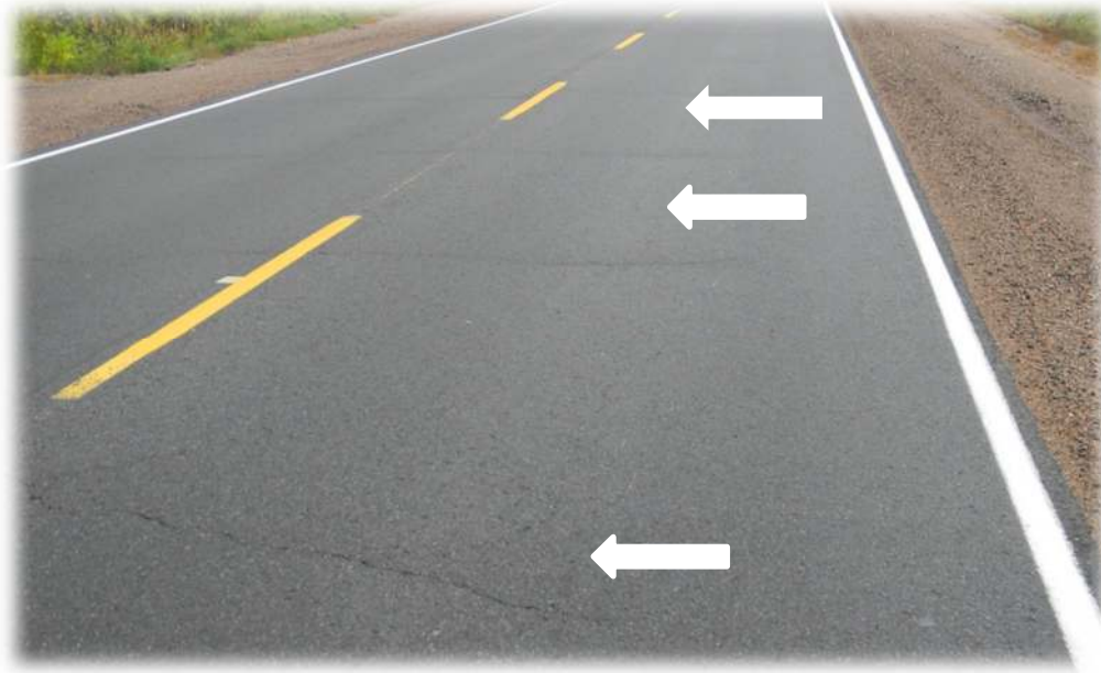
Figure 8: Reflective Transverse Cracking on Newer Pavement
