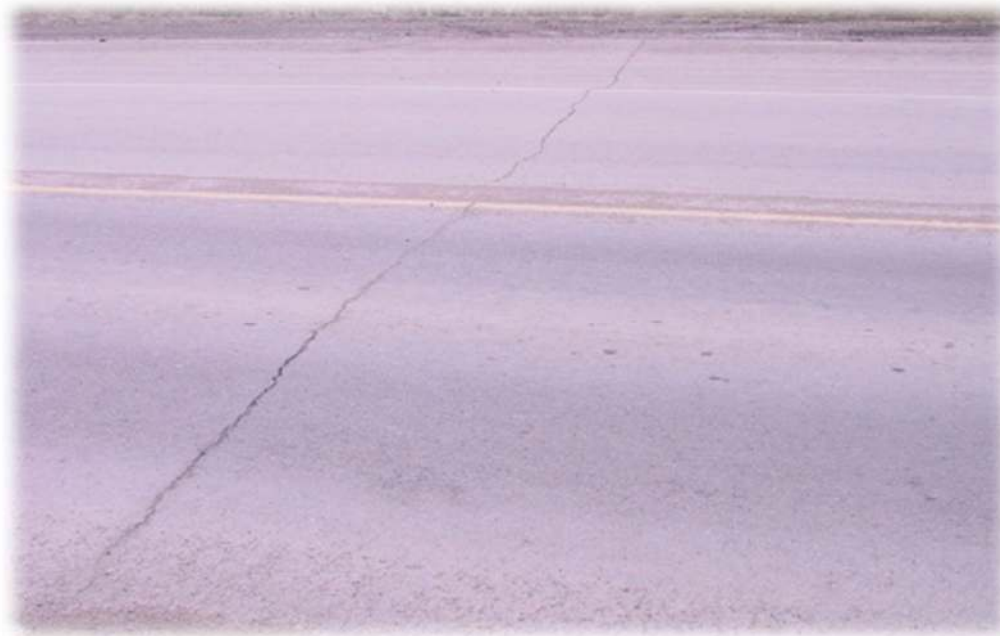
Figure 7: Transverse /Thermal Cracking (Non Structural)
