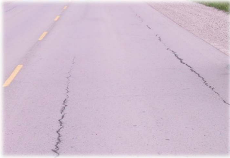
Figure 3: Wheelpath Fatigue Cracking
