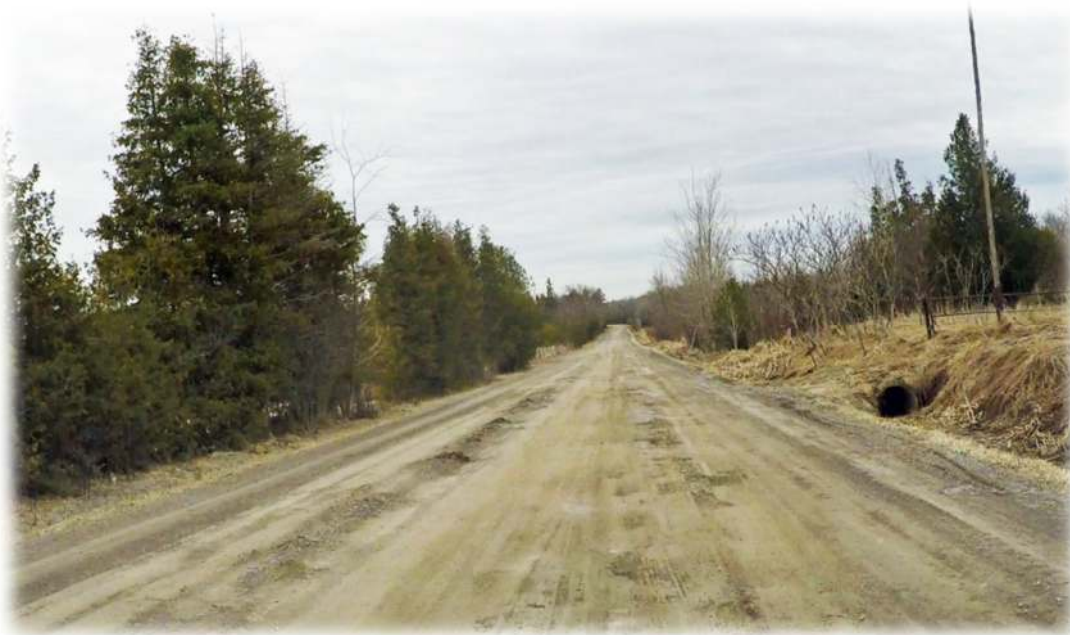
Figure 2: Structurally Inadequate Low Volume Road
