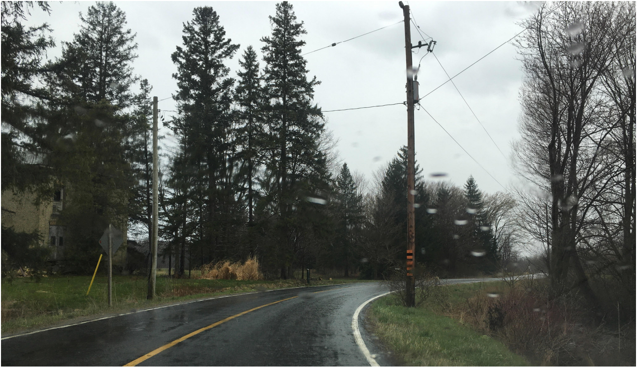
Dingle Street - Hazard sign blocked by vegetation
