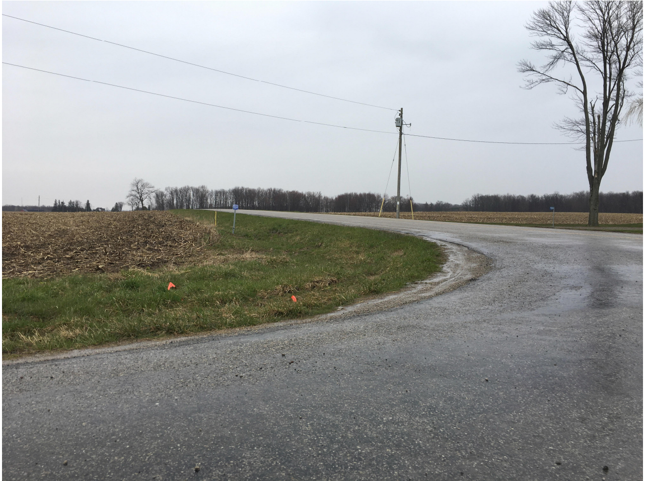
Van Patter Line – Intersection with Hacienda Road facing north. 80m sightline for southbound Hacienda Road traffic.
