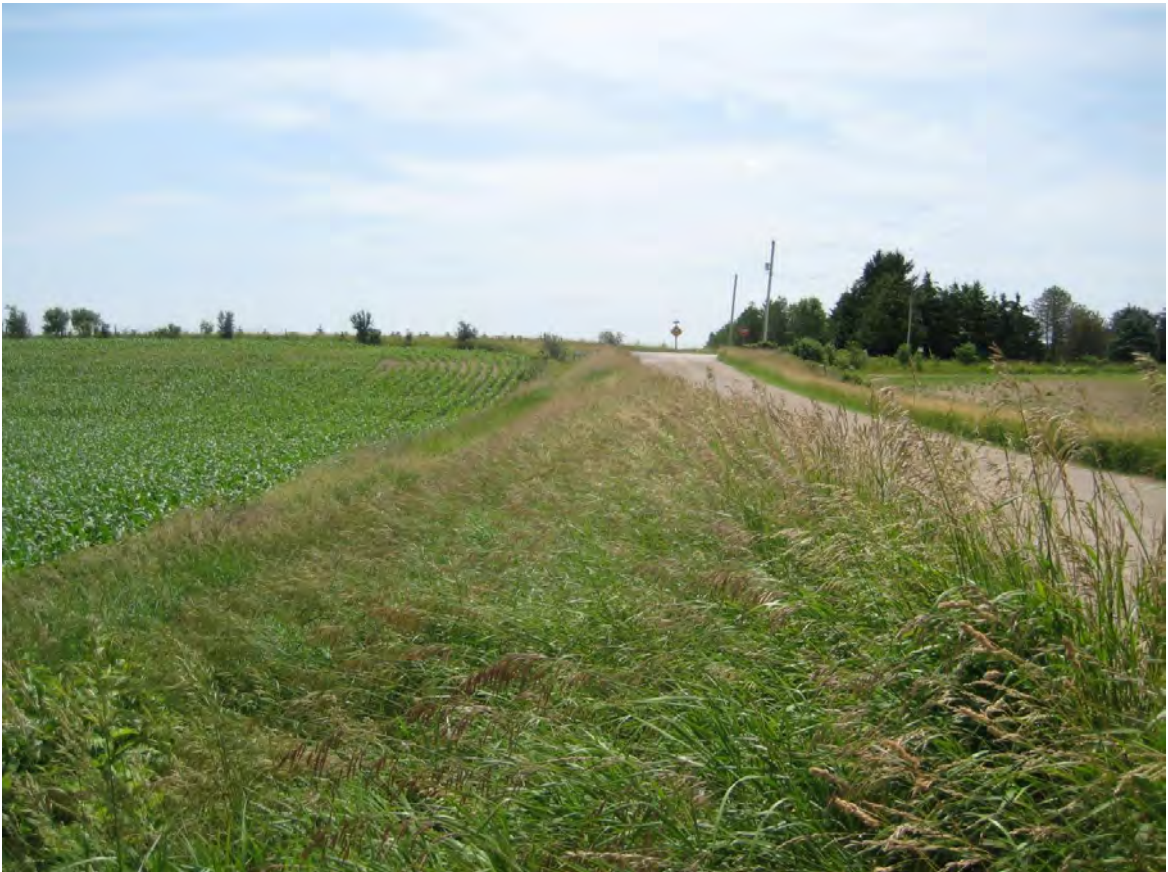
Helder Road – Ditch within clear zone, on east side, facing Yorke Line intersection.
