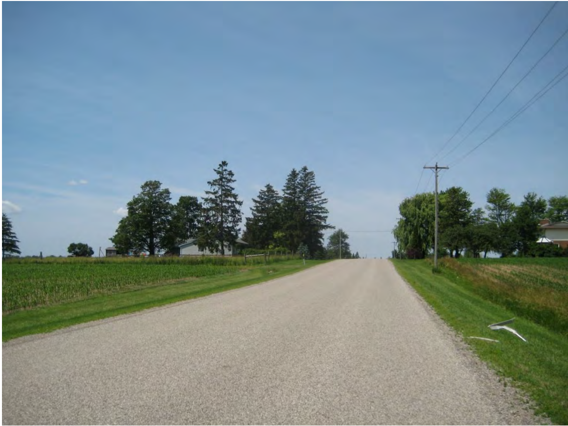
Wilson Line – Poor visibility due to vertical alignment.
