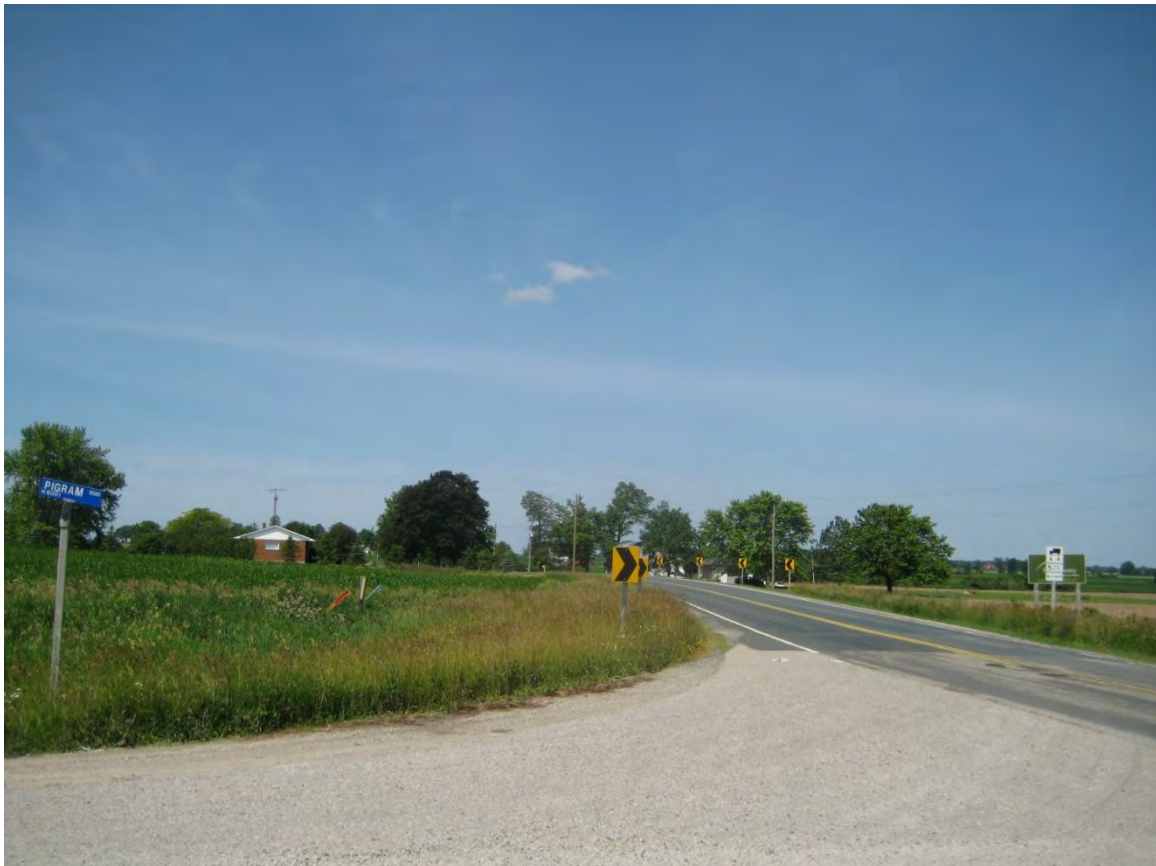
Pigram Line – Poor visibility facing east at Avon intersection due to horizontal alignment.
