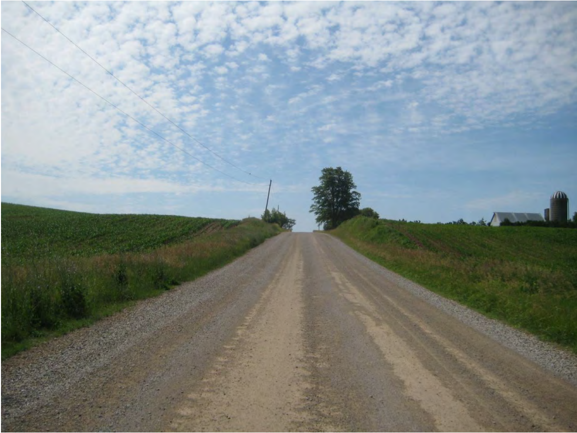
Pigram Line – Poor visibility approaching Wilson Line intersection from north.
