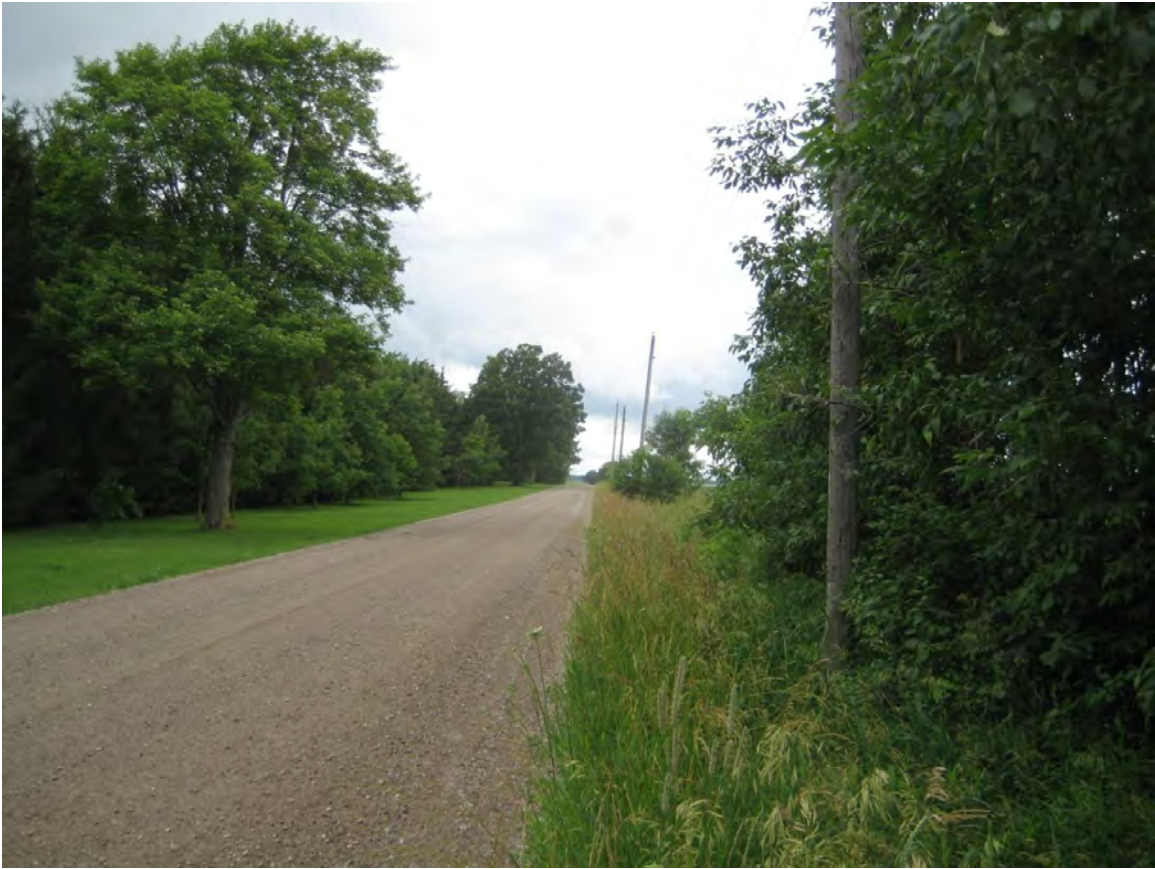
Newell Road – Hydro pole and ditch within clear zone (north of Ron McNeil Line)
