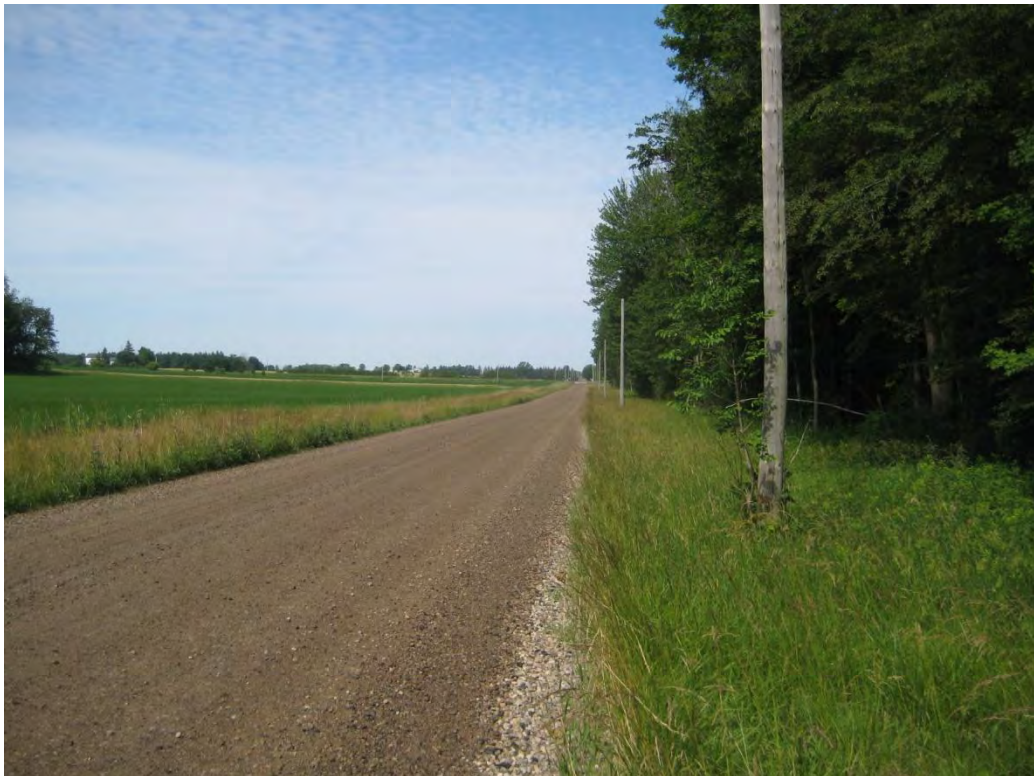
Crossley Hunter Line – Hydro poles within clear zone on north side (facing west), west of municipal number 51986.
