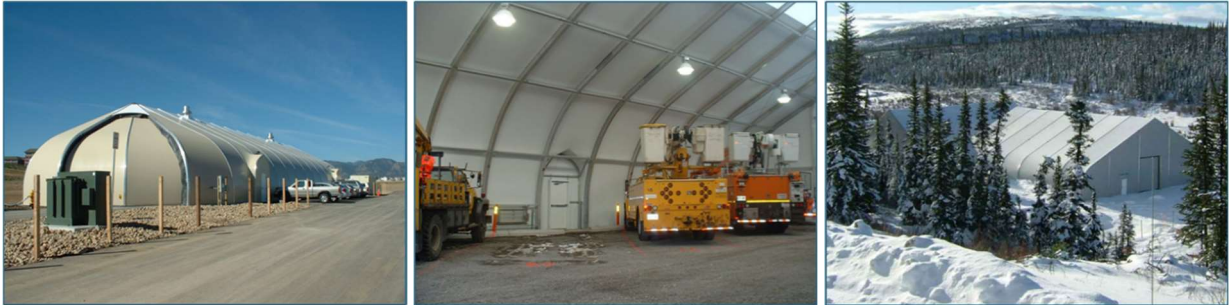
Figure 25 - Examples of Public Work Yard with membrane construction
